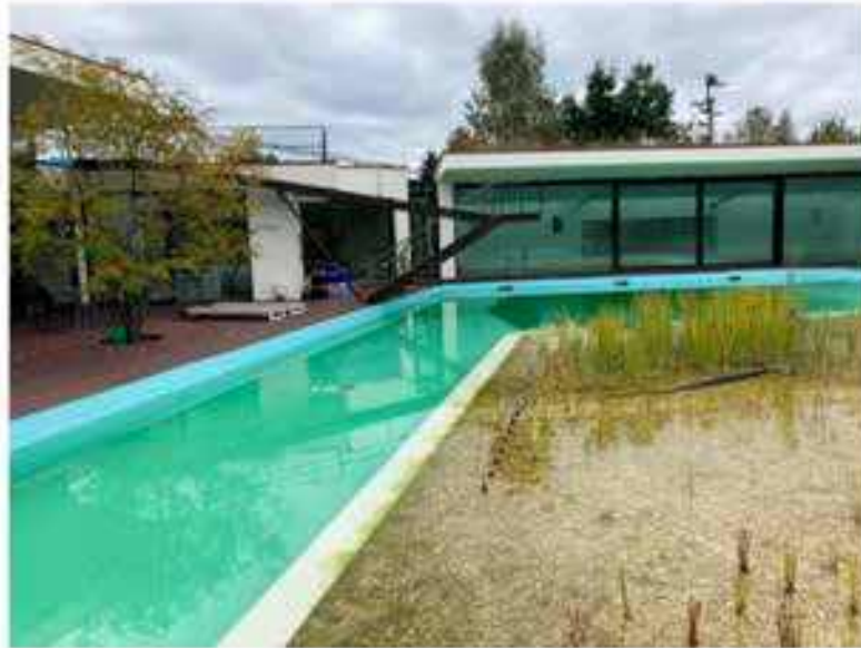
Figure 8. Swimming pond with a regeneration zone and accelerated mineral filtration (photo by W. Walczak).
