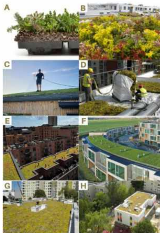
Fig. 1. A. A green roof module constructed from a tray; B. Plants used; C. Maintenance process; D. Installation of modular green roof; E. Carlsberg Byen district of Copenhagen ( https://www.shl.dk/work/dahlerups-tower?utm_source ); F. Nye district of Aarhus N, Denmark ( https://www.designboom.com/architecture/big-modular-housing-spirals-pond-danish-sustainable-suburb-09-29-2022/?utm_source ); G. 3A Wyzalazek Street in Warsaw, Poland; H. A Baluty nursery school in Warsaw, Poland ( https://stelone-budownictwo.pl/ ) (date of access: 4 July 2025); www.natureimpact.com (date of access: 4 July 2025).
