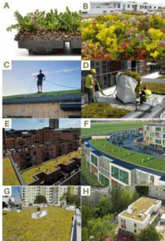
Fig. 1. A. A green roof module constructed from a tray; B. Plants used; C. Maintenance process; D. Installation of modular green roof; E. Carlsberg Byen district of Copenhagen ( https://www.sbl.dk/work/dahlerups-tower?utm_source ); F. Nye district of Aarhus N, Denmark ( https://www.designboom.com/architecture/big-modular-housing-spirals-pond-danish-sustainable-suburb-09-29-2022/?utm_source ); G. 3A Wyzalazek Street in Warsaw, Poland; H. A Baluty nursery school in Warsaw, Poland ( https://stelone-budownictwo.pl/ (date of access: 4 July 2025); www.natureimpact.com (date of access: 4 July 2025)).
