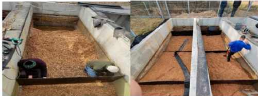
Figure 6. Photos of filter during montage of walls.
