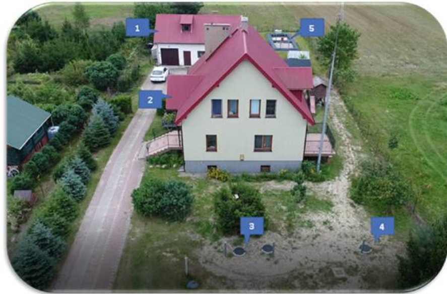
Figure 2. Employee housing unit in Kulczyn, Polesie National Park—location of facilities on the plot: 1—outbuilding; 2—residential building; 3—primary settling tank; 4—pumping station; 5—hybrid constructed wetland integrated into a closed water circuit (photo by Radomir Obroślak).
