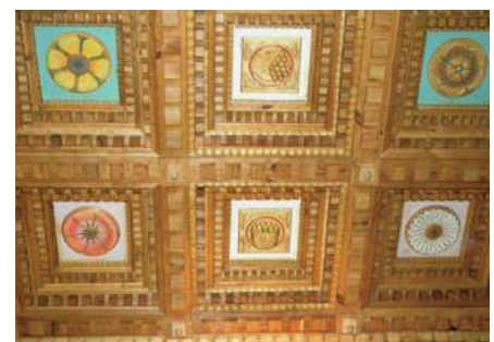
Photo 12.28. Coffers on the ceilings in the church in Momoty Górne. Source: Bahej 2009.
