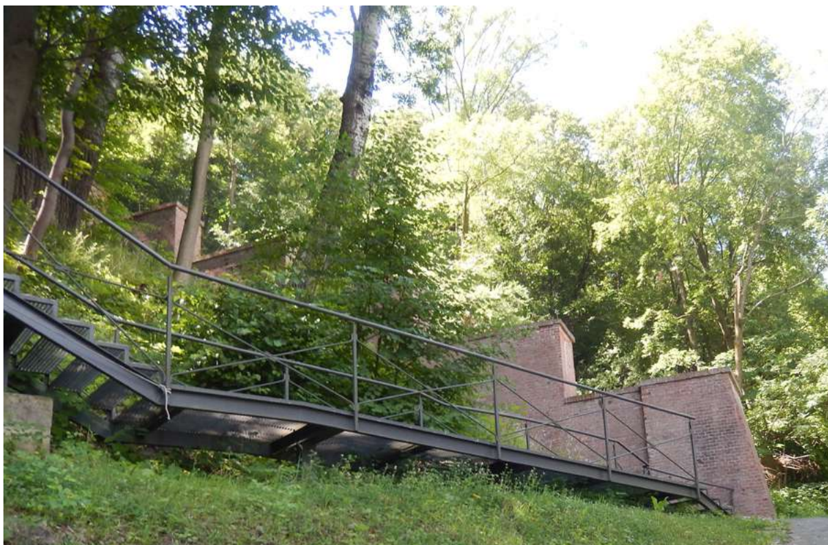
Photo 13.13. Elevation above the Sanok Gate. Photo by Anna Mazurek-Kusiak
