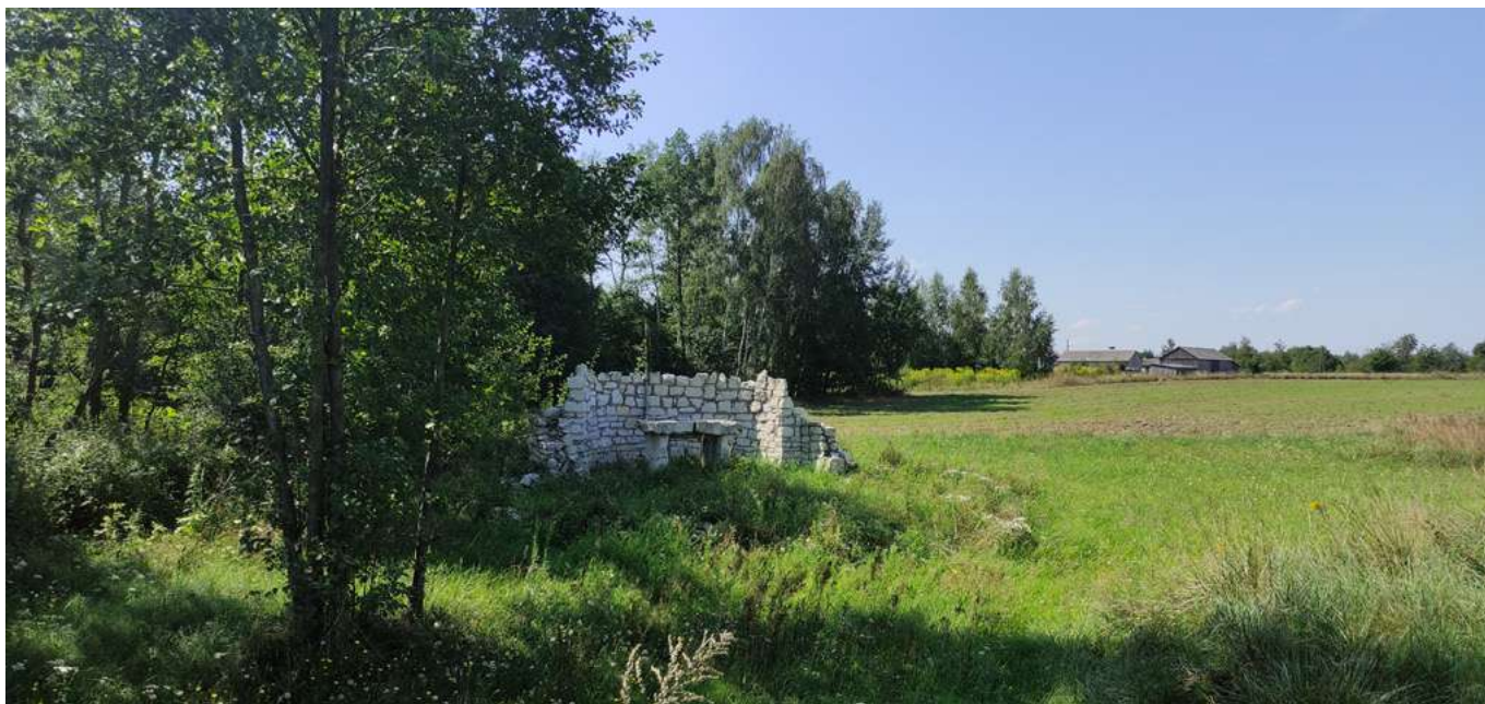
Photo 7.3. Foundations of the Romanesque chapel. Photo by Agata Kobyłka
